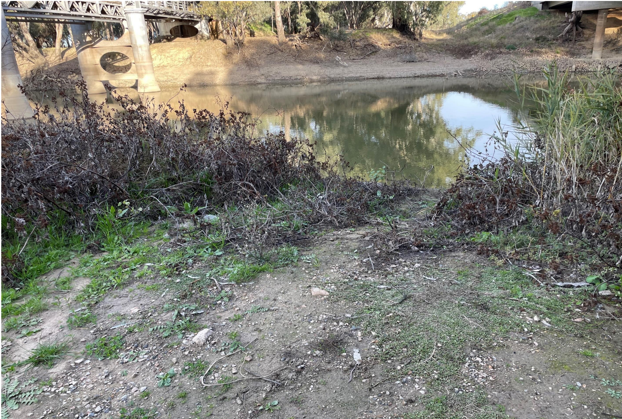
Water entry; excavation of high points to establish even grade on approach to water. Grade compliant with NSW Boat Ramp Facility Guidelines. (See construction design plan details for particulars)
