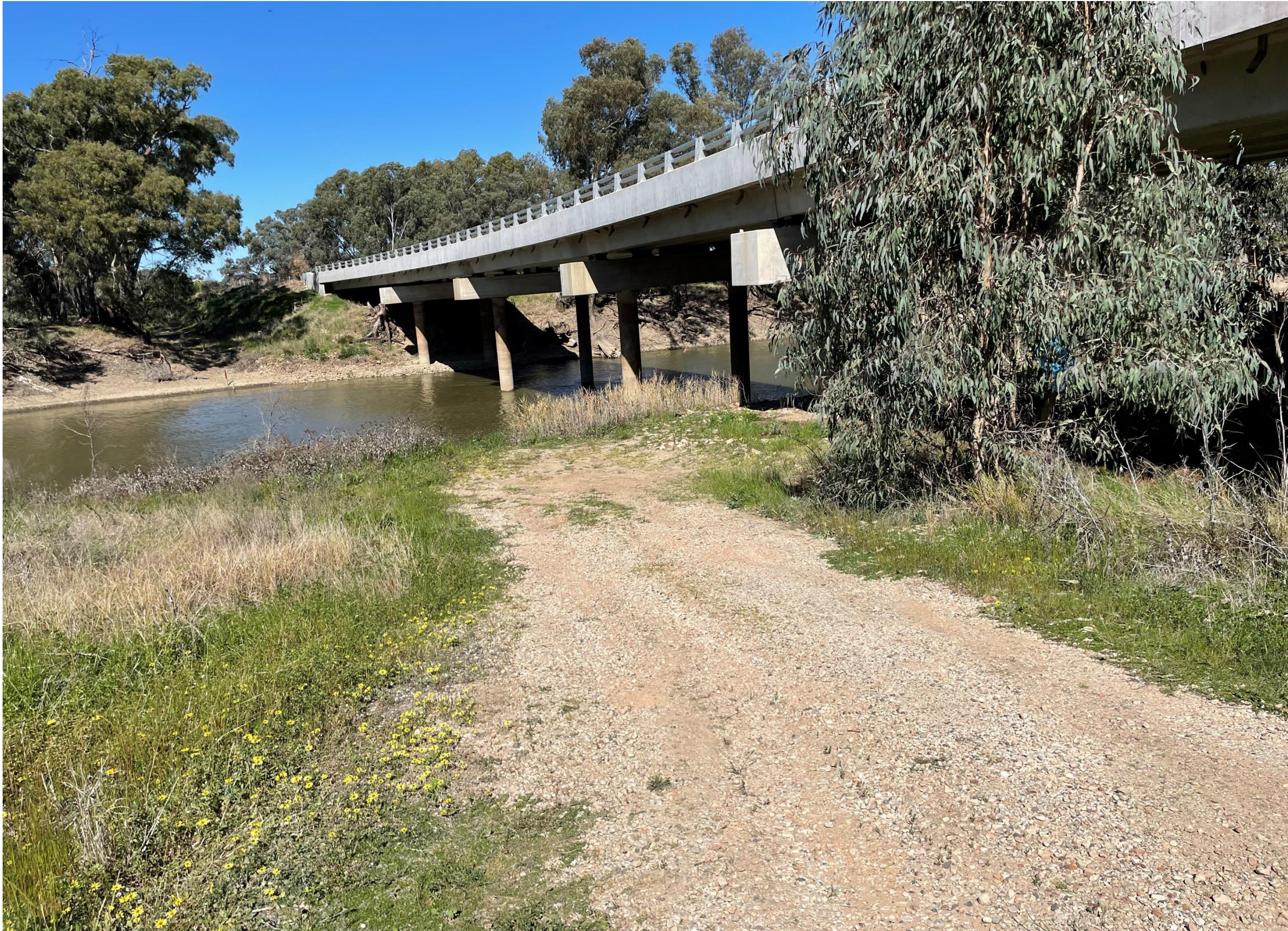
Existing pavement to have gravel added, trimmed and resealed to the lower terrace. (See construction plans for dimensions; 4m past the eucalypt tree)
