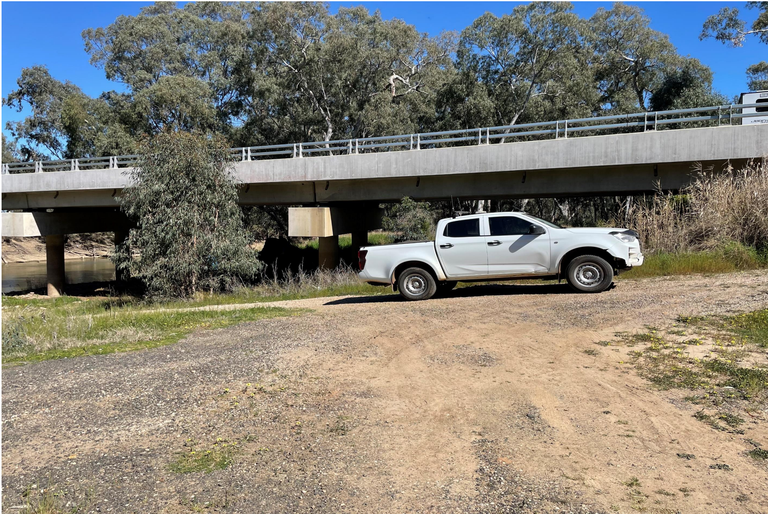
Vehicle on boat ramp approach to waterline. The former bridge construction track to be recompacted and trimmed for sealing to ensure no erosion. Concrete matting to be used as boat ramp surface on immediate approach to water for a substantial structure to cater for increased flows and higher river levels.
